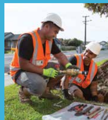
Servicemen Wesley Sio and Tafunai Olo don Watercare-branded high-visibility vests with their ID cards visible while connecting a water meter.
